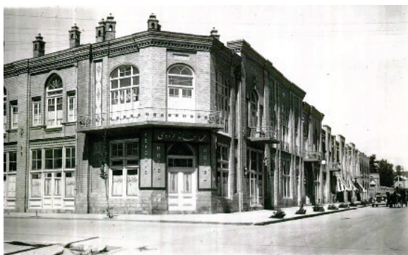
Figure 8. Firdausi Hotel, under construction, ca. 1935–36. Source: Estādūx
